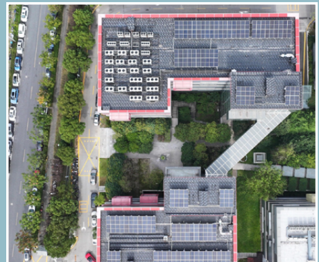
Zhangjiang Data Center in Shanghai
